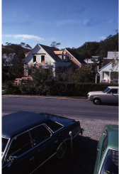
36 Commercial Street (home of Lauren Richmond and Bruce Deely) undergoing renovation in 1977
