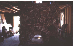
36 Commercial Street - renovation in 1977 Conrad Mallicoal living room fireplace - nearing completion
