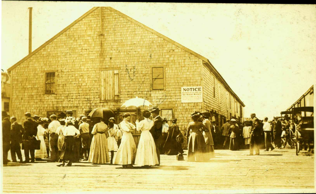
END OF WHARF
