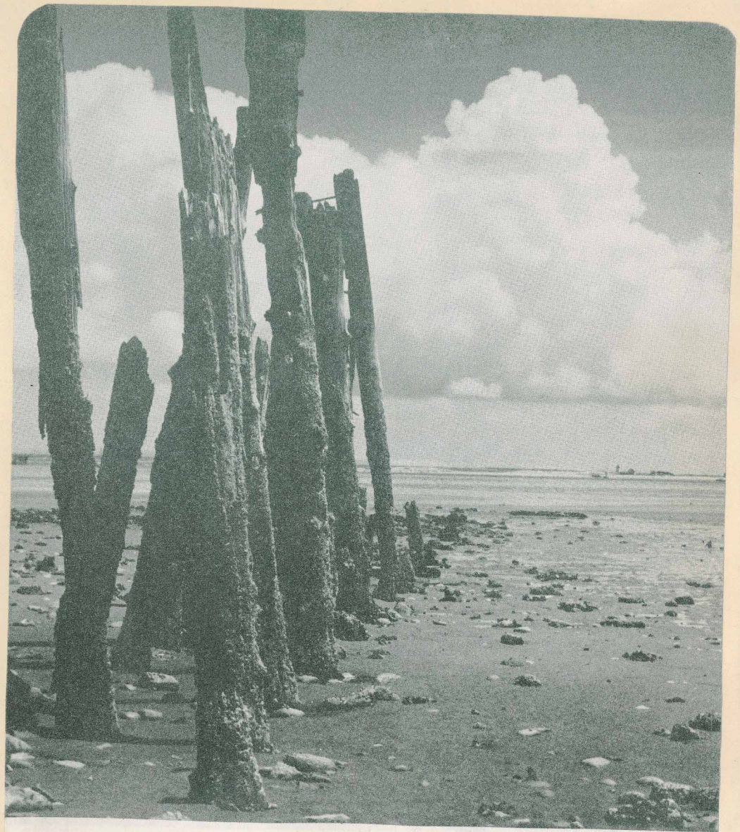
EBB TIDE - Long Point, Right - 1954 - John W. Gregory The ancient piles of an old wharf stand starkly silhouetted against the sky.
