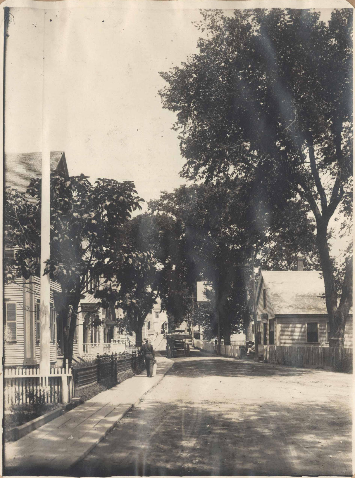
Another view facing east. Duarte's Shoe Shop, right - 1900
